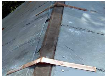
Fig 1. Screw or nail the copper fixing straps to your roof tiles at approximately 400 - 600mm centres.
